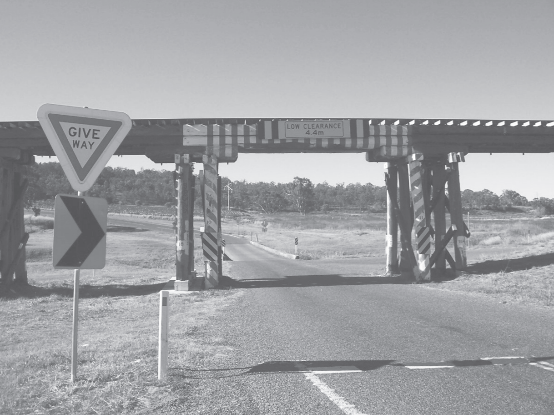
The railway underpass and single lane bridge section of the soon to be re-zoned Warwick-Allora road.
