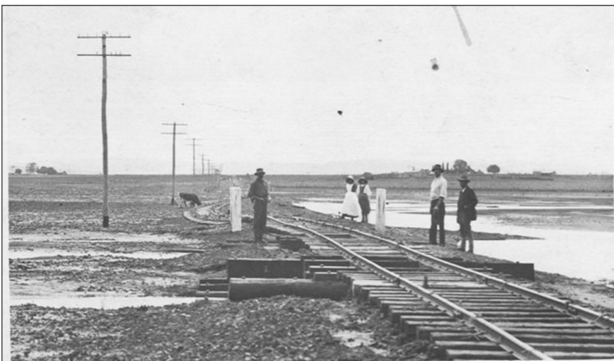
The above photos are taken circa 1917. Both are taken from Hendon looking towards Allora. TOP: Floodwater over the "Log Road" and ABOVE: Flood damage to the railway line.
