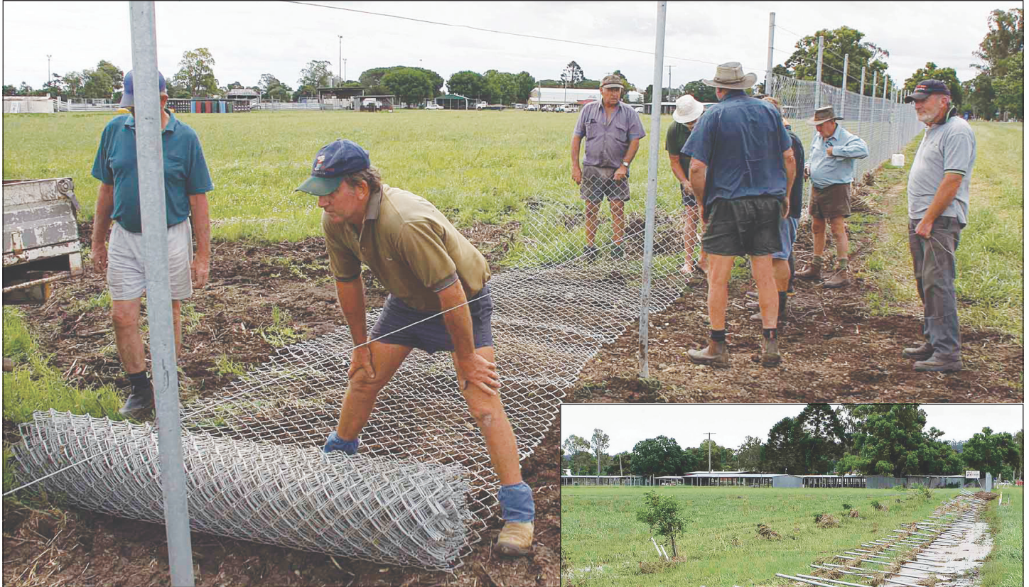
ABOVE: Within hours of starting work, the repair team had the site cleared and the poles back upright. The first roll of chain link is rolled out and attached to the undamaged part of the fence.
