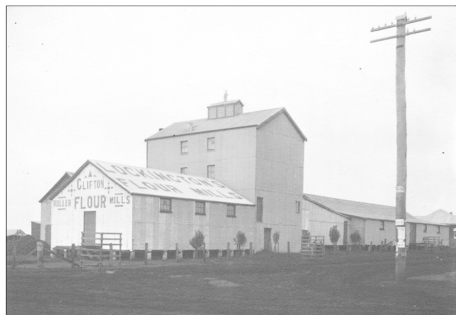
Clifton flour mill destroyed by fire in January 1912
