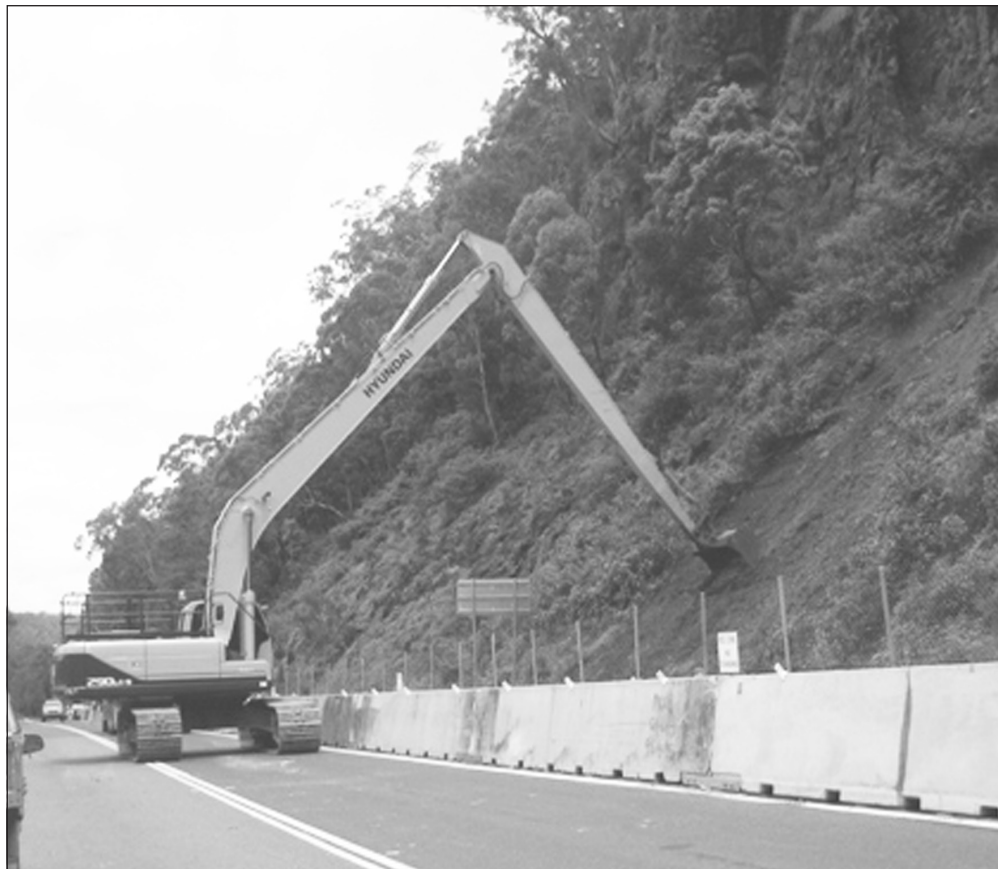
LEFT: Cunninghams Gap slope remediation
