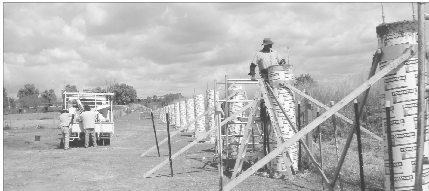
Building the new pillars for the sewer main from the industrial estate in Kenilworth Street, Warwick.
