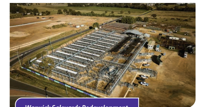
Warwick Saleyards Redevelopment
