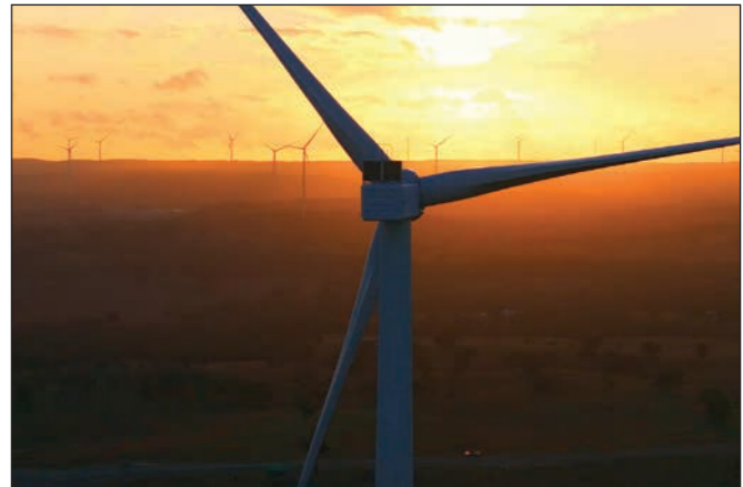
The enormous MacIntyre Wind Farm, south of Karara, has recently begun pumping power into the national grid.
