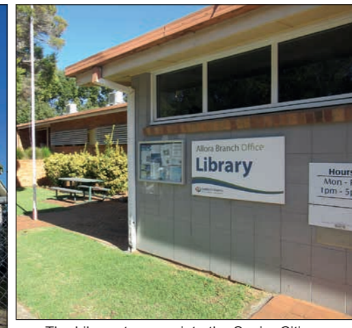
The Library to move into the Senior Citizens Building and the Sports Museum to expand into the Library - this corner block of buildings will be known as Allora's Community Precinct.
