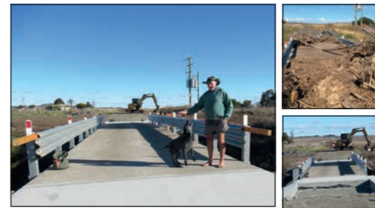
TOP RIGHT: Kital Road Bridge in 2022 and ABOVE RIGHT: 2023.
