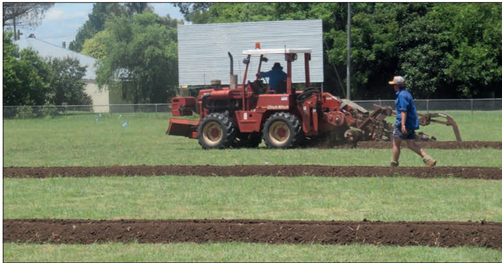
Preparing the oval for laying the irrigation pipes.
