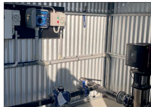
LEFT: Inside the pumping station shed.
