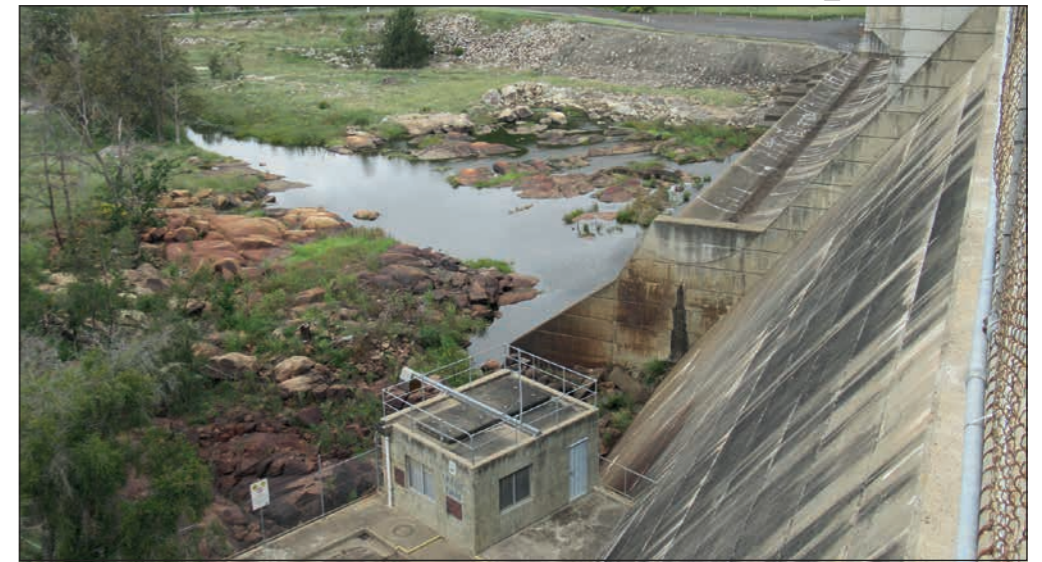
Pump Station at Leslie Dam.
