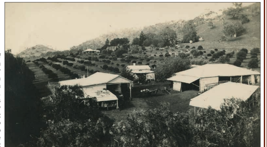
The packing shed (left), outbuildings, and part of the orchard at Belle Vue, Goomburra.
