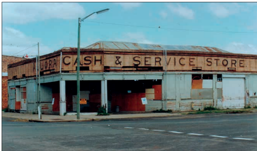
The demolition of the old Barnes & Co/Allora Motors building.
