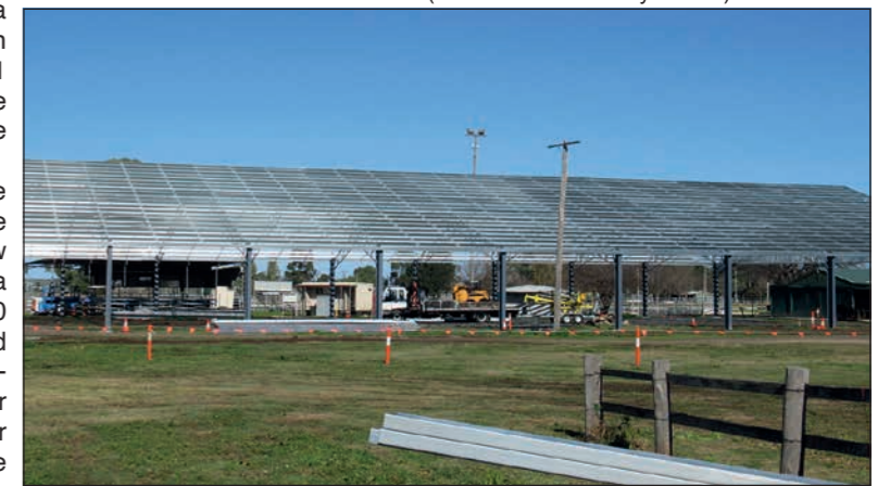
to here... (Arena taking shape.)
