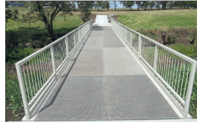
A highlight of Lenny's year as President was the building of the Maher-Rickert Bridge across the Dalrymple Creek on the Allora Golf Course.
