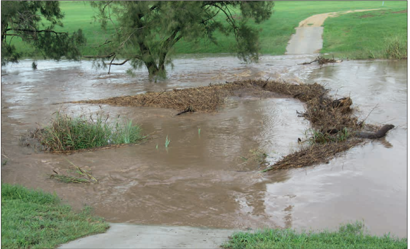
The Maher-Rickert Bridge stood the big test when the Dalrymple Creek flooded and completely submersed the bridge covering it in water, debris and some rats.
