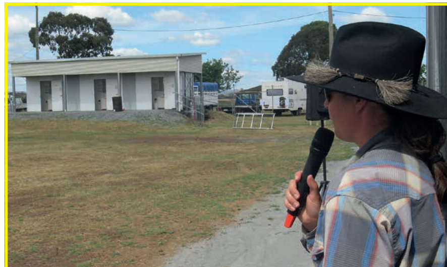
Stud Cattle Chief Steward Melinda Hoey with the newly constructed amenities block in the background.
