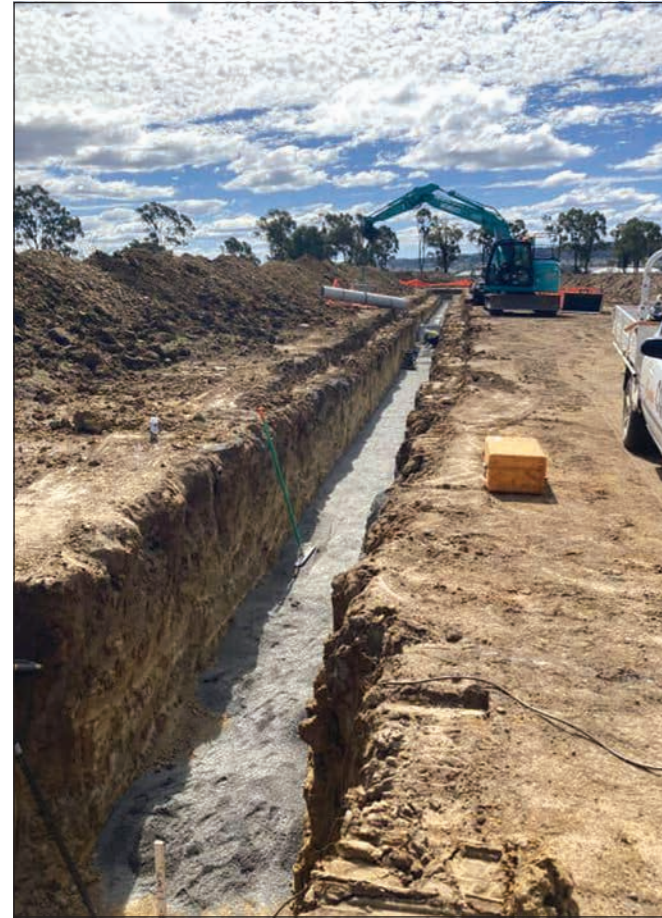
Coops equipment working on a sub-division in Warwick.
