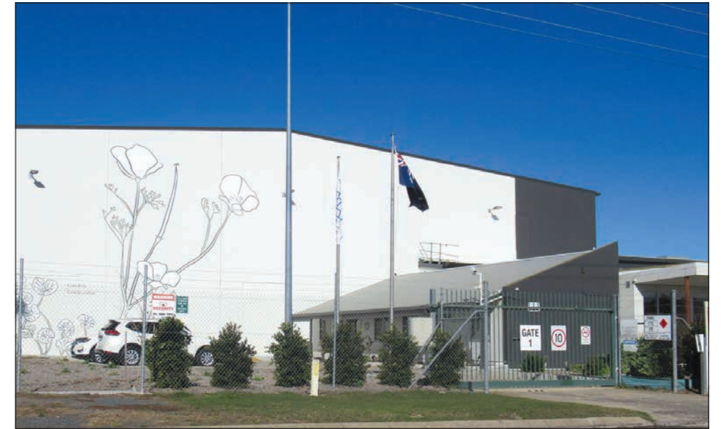
Integria's expanded production facility in Warwick.
