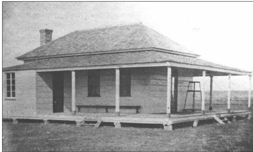
Allora's first Town Hall built in Forde Street in 1870.
