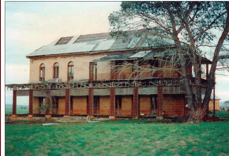
Glengallan Homestead taken in 1993 before the restoration.
