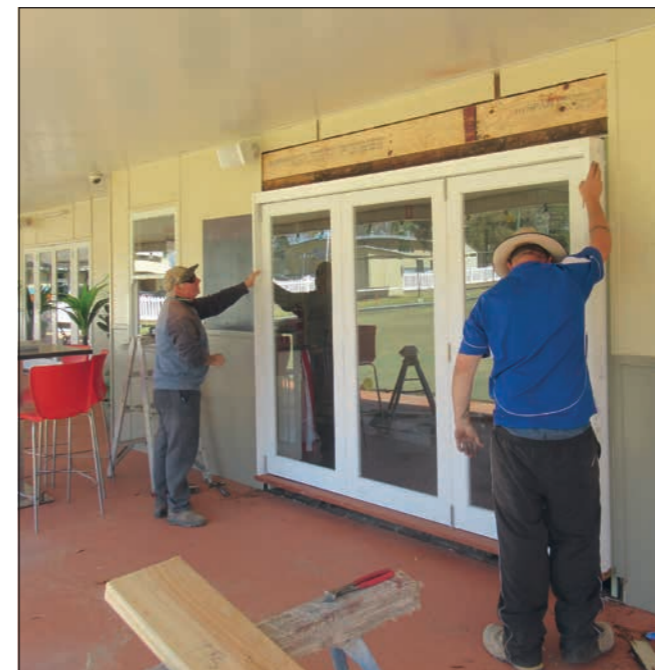
Richard Kyle and Joel Merryl replacing the doors.
