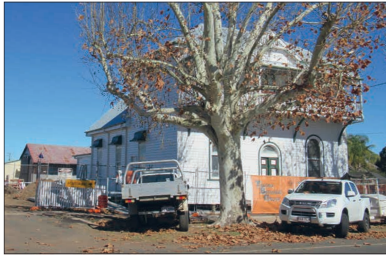
Restoration currently underway at the Old Shire chambers.
