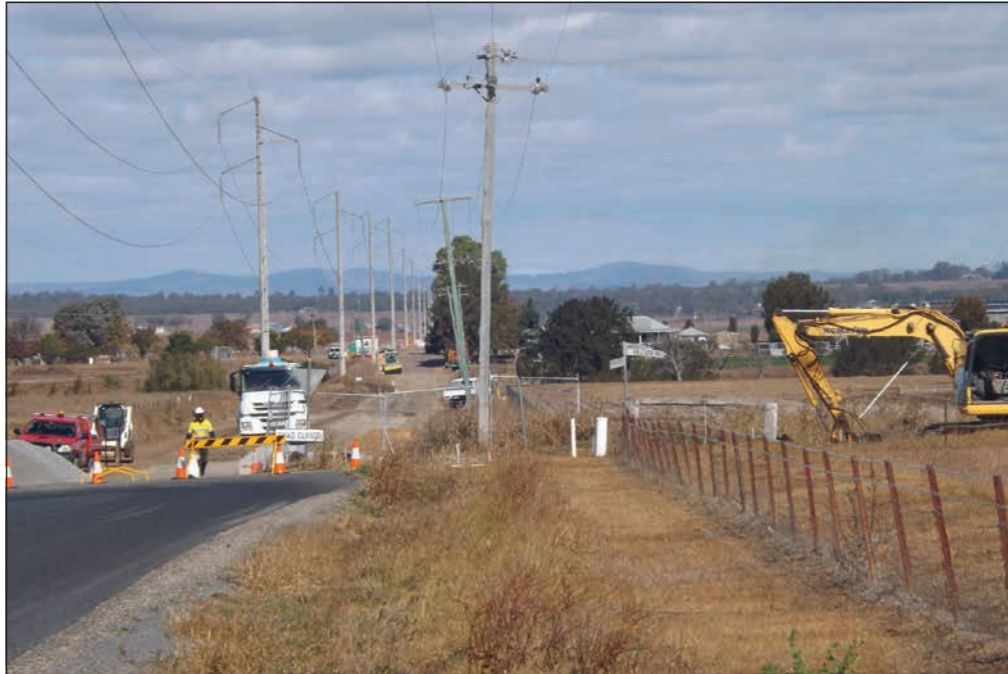
Roadwork underway on Merivale Street, Allora.
