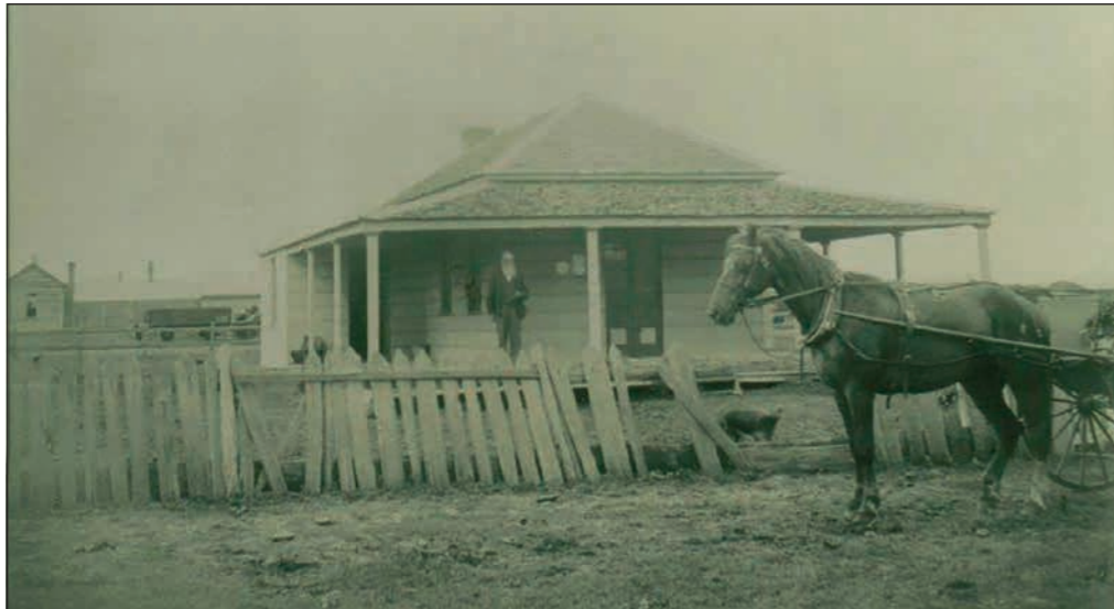
Allora's first Town Hall built on site now occupied by the Allora & District Historical Society. The building which faced Forde Street was built by James Dougall for a cost of One Hundred and Eighty Four pounds in 1870. It measured 35 feet by 18 feet with a main room and two ante rooms. The hardwood timber was sawn out by hand. The pine came from Highfields.
