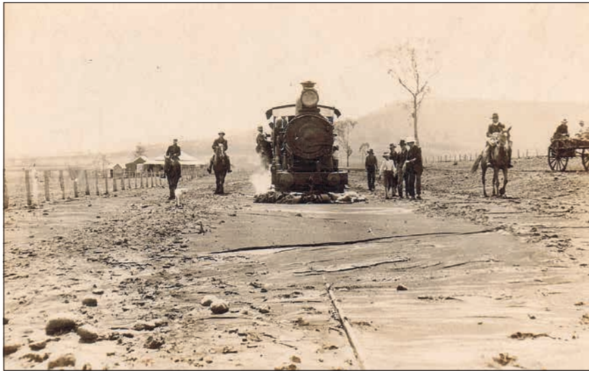
The Goomburra train bogged in silt over the line at Kunda.
