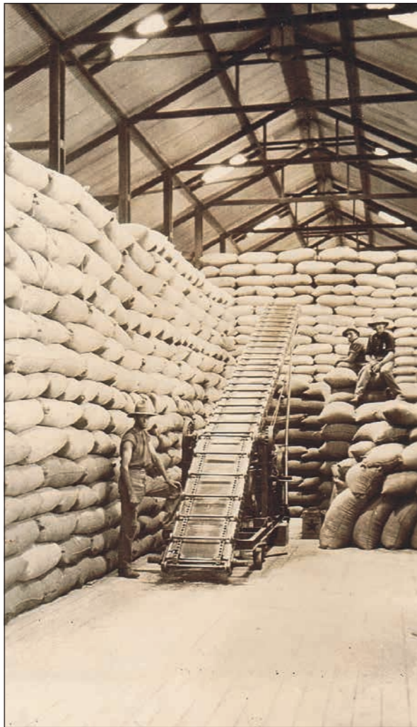
Inside the Allora grain shed (now Jenco) in 1927. George Ellis senior is standing at the end of the elevator. accepted in Allora by the State Wheat Board in the 1968 season)
