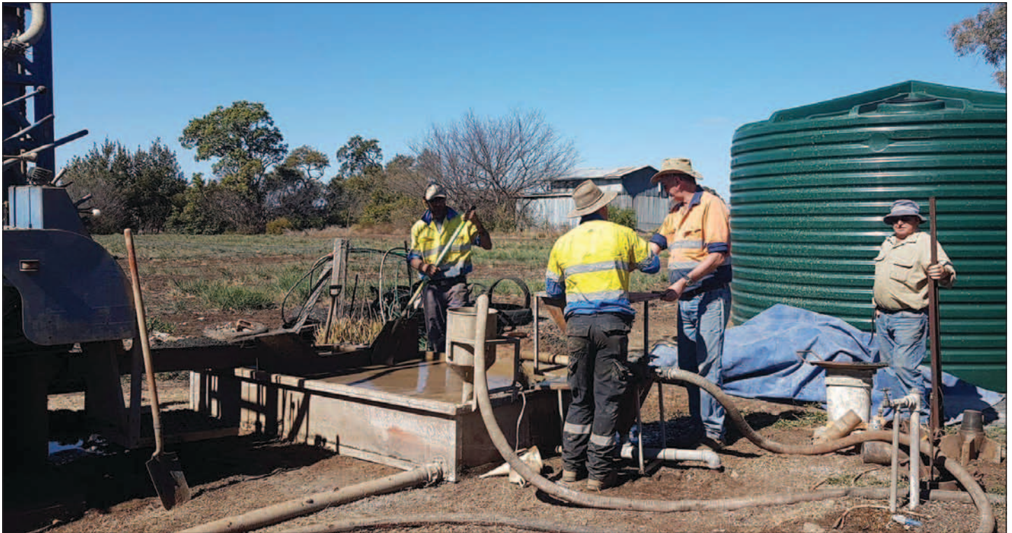
Drilling success - Water for Allora Mulberry project tapped.
