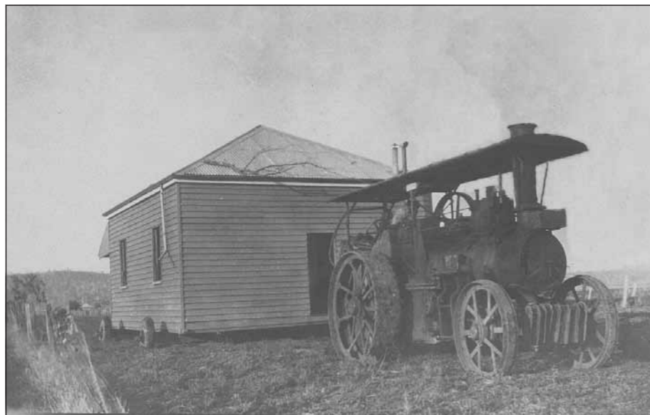
Bill Doyle's traction engine shifting a house in the Allora district.
