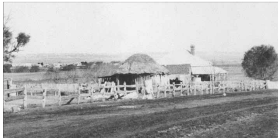
Stallman's house on the Allora-Clifton Road in 1897.
