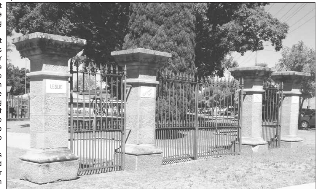
The Glengallan Gates located in Leslie Park, Warwick
