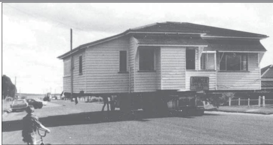
The former Allora State School residence being moved from Warwick Street to Gordon Street by the Allora Hospital Board for use by the Allora Community Kindergarten Association.
