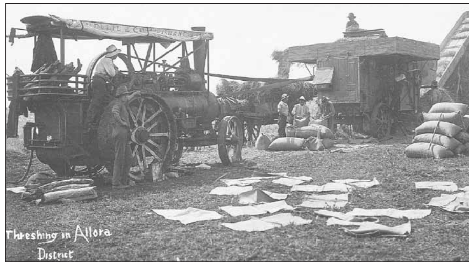
A wheat threshing plant in the Allora district.
