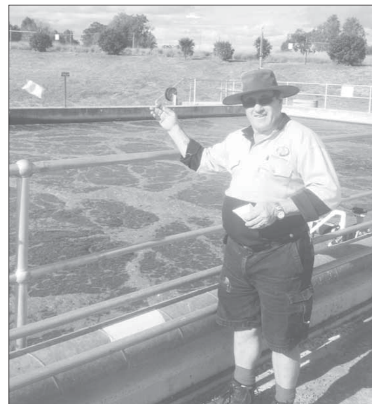
SDRC's Wastewater Treatment Operator Derrick Zwoerner adds an Eco-tab to the WWTP.
