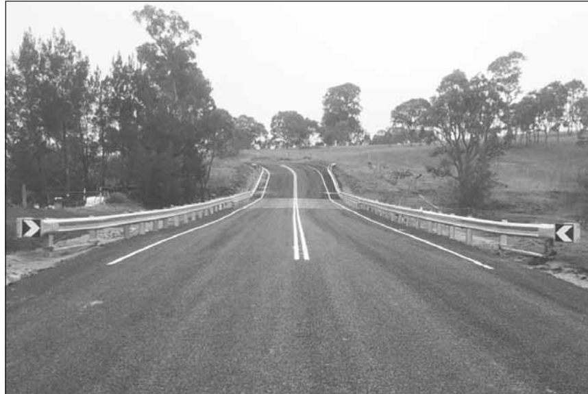
Bellinghams Road Bridge.
