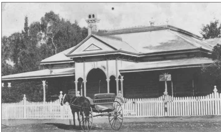
The Queensland National Bank, Drayton Street, Allora.
