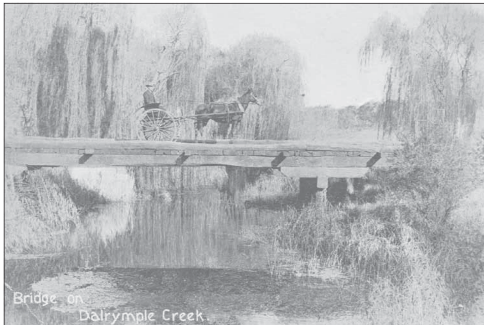
The bridge over Dalrymple Creek.
