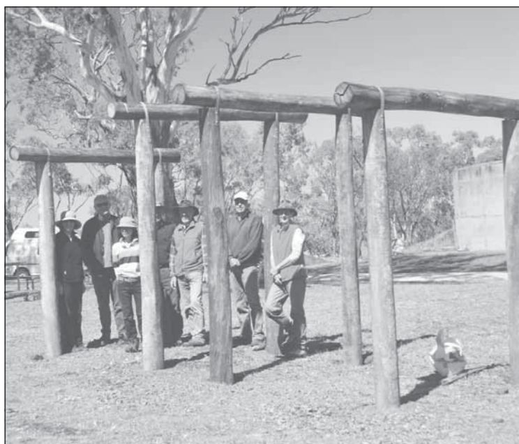
Allora Landcare Group members at the framework for the new shed.
