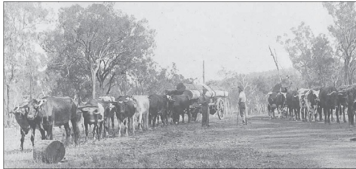
No photos of Gordon's sawmills at Allora or Goomburra were available for printing this week. Instead, pictured here is Bill Springate's bullock team hauling logs on the Pratten road. Bill Springate is on the left, in front of wagon.
