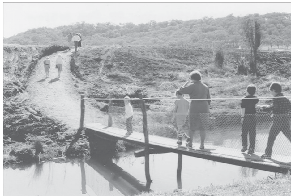
Temporary bridge over Dalrymple Creek. "Back to Allora" Day 1988.
