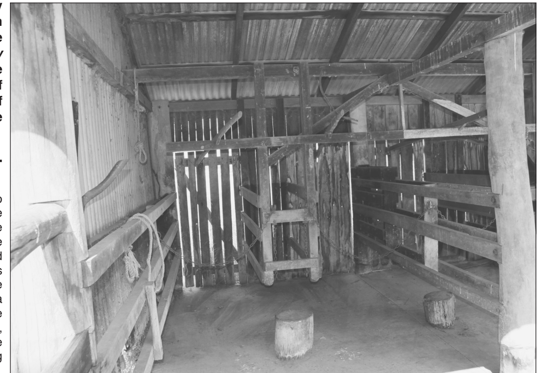
Milking stalls in the 3 bail dairy at Dalrymple Creek.
