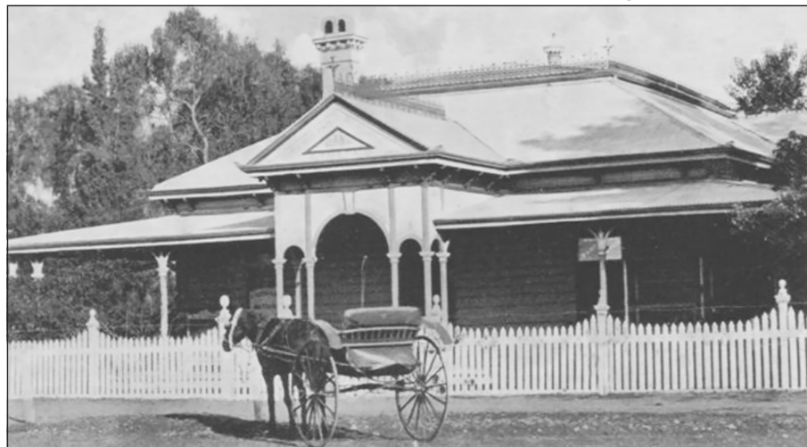
Queensland National Bank, Drayton Street, Allora, circa 1905.
