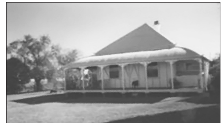
Mr. and Mrs. Charles Burge's house shifted from Allora-Clifton Road to Mt. Marshall
