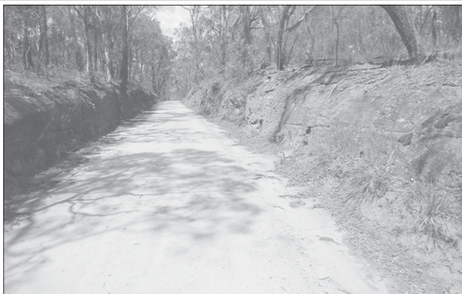
Sandstone cutting on Yankee Gully Road
