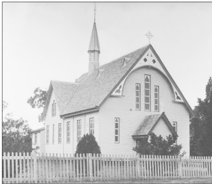
St. David's Church with the original shingle roof.
