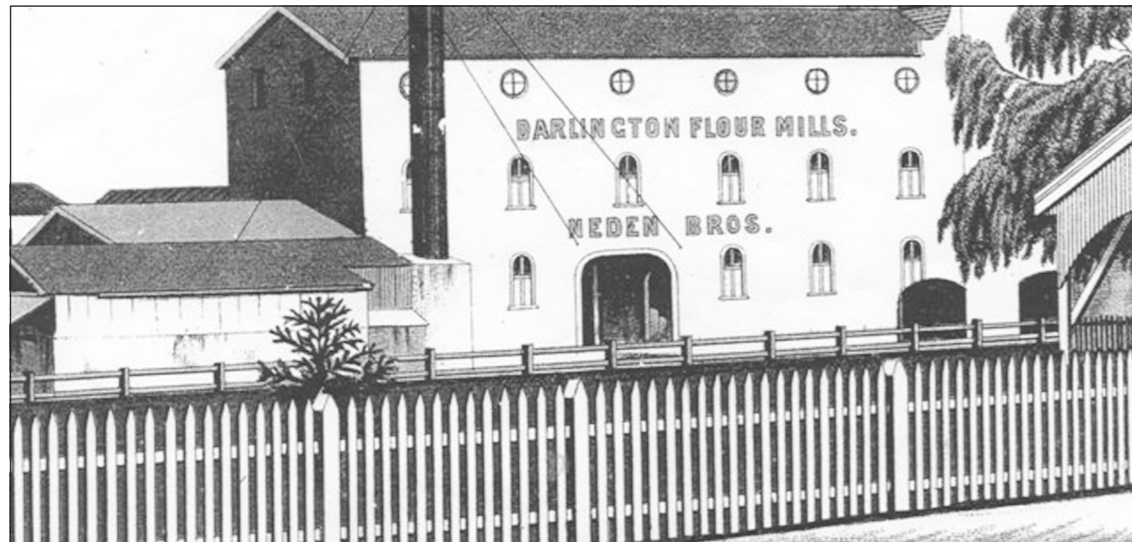
Darlington Flour Mill, Toowoomba. Photo courtesy Rod Gisler
