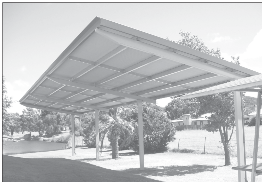
LEFT: The new structures at Stanthorpe skate park.
