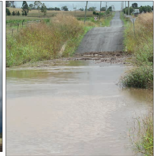
Merivale Road crossing, Allora.
