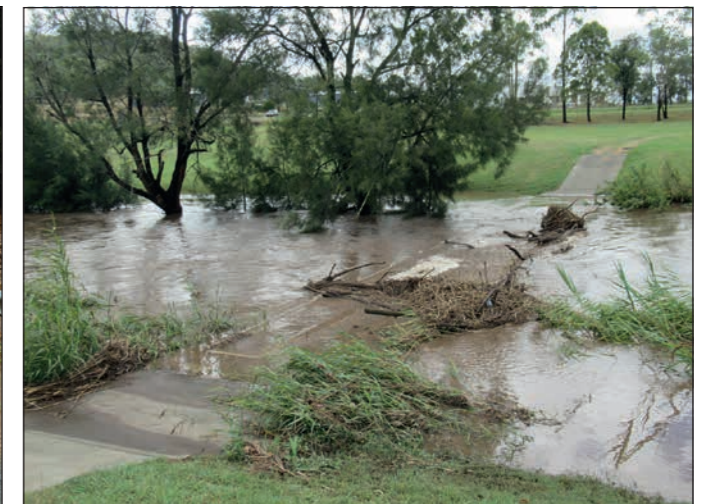
Allora Golf Course Maher Rickert bridge.
