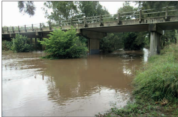
New England Highway bridge.
